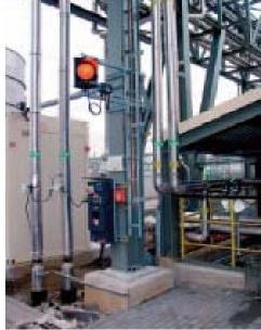
Armored cable in protected raceways are used to keep a clean appearance and when cable tray runs are not practical....
